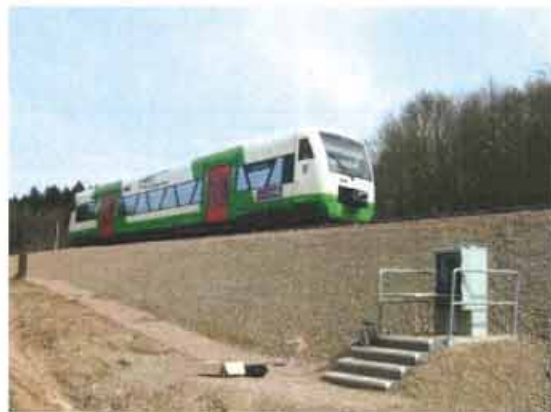
Fig.2 Outdoor housing of the measuring units
